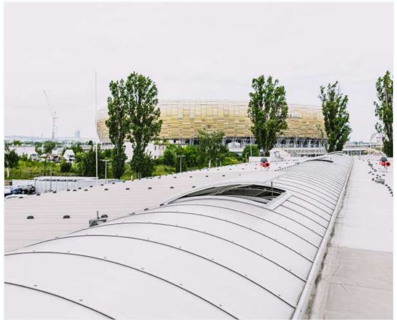
Fig. 1 – mcr PROLIGHT continuous rooflight with open vent
