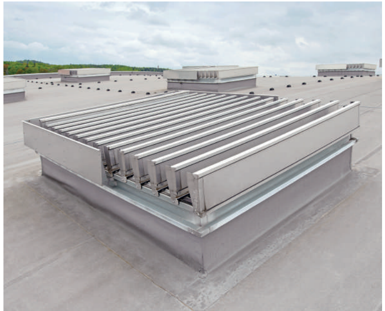
Fig. 37 – mcr LAM louvered vent, roof mounted
