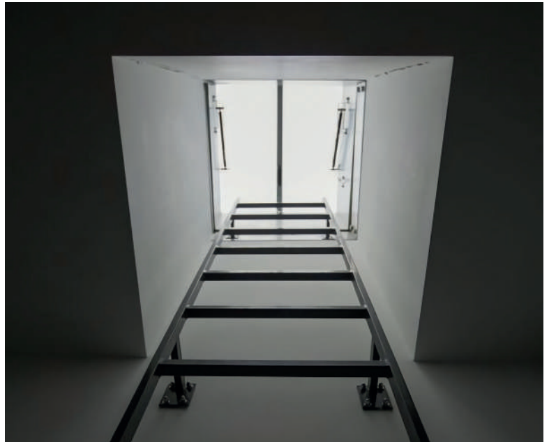
Fig. 13 – mcr PROLIGHT roof hatch
